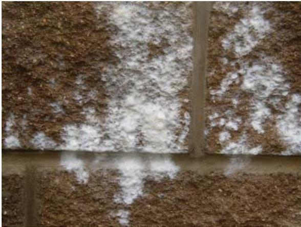
An example of efflorescence caused by calcium chloride in concrete.
